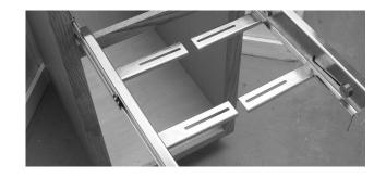
**Step 6.** With both slides full closed and inside the cabinet, apply the double-sided tape to the front of the slide flanges.
