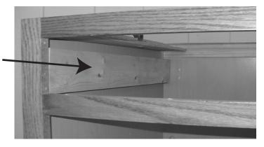
Step 3. Mark the location of the front mounting hole by measuring UP 13/4" from the LOWEST point of your opening and BACK 1/4" from the front of the opening. Once marked install slides to side of cabinet insuring they are level.
